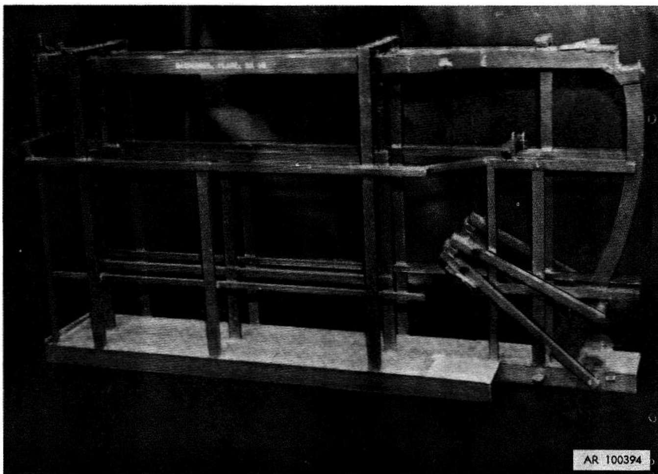
Figure 1-5. Dispenser assembly of flare dispenser XM19- snout retracted.
