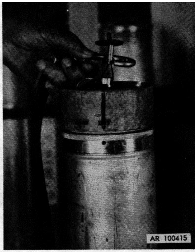
Figure 2-16. Attaching static line XM164 to pull cable assembly
